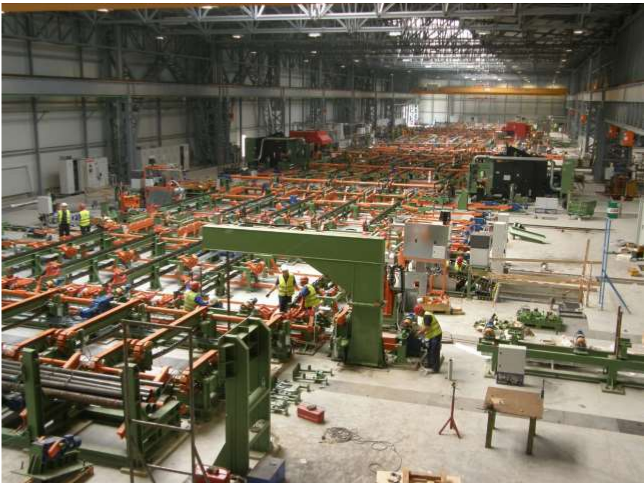
Threading and phosphating OCTG premium line for tubes dia. 60 -180 mm – During the erection
