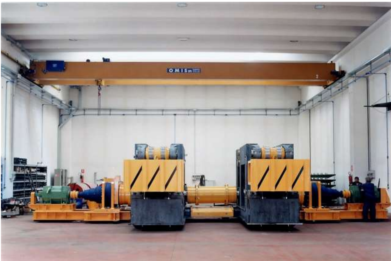
Charging pushers for billets reheating furnace
