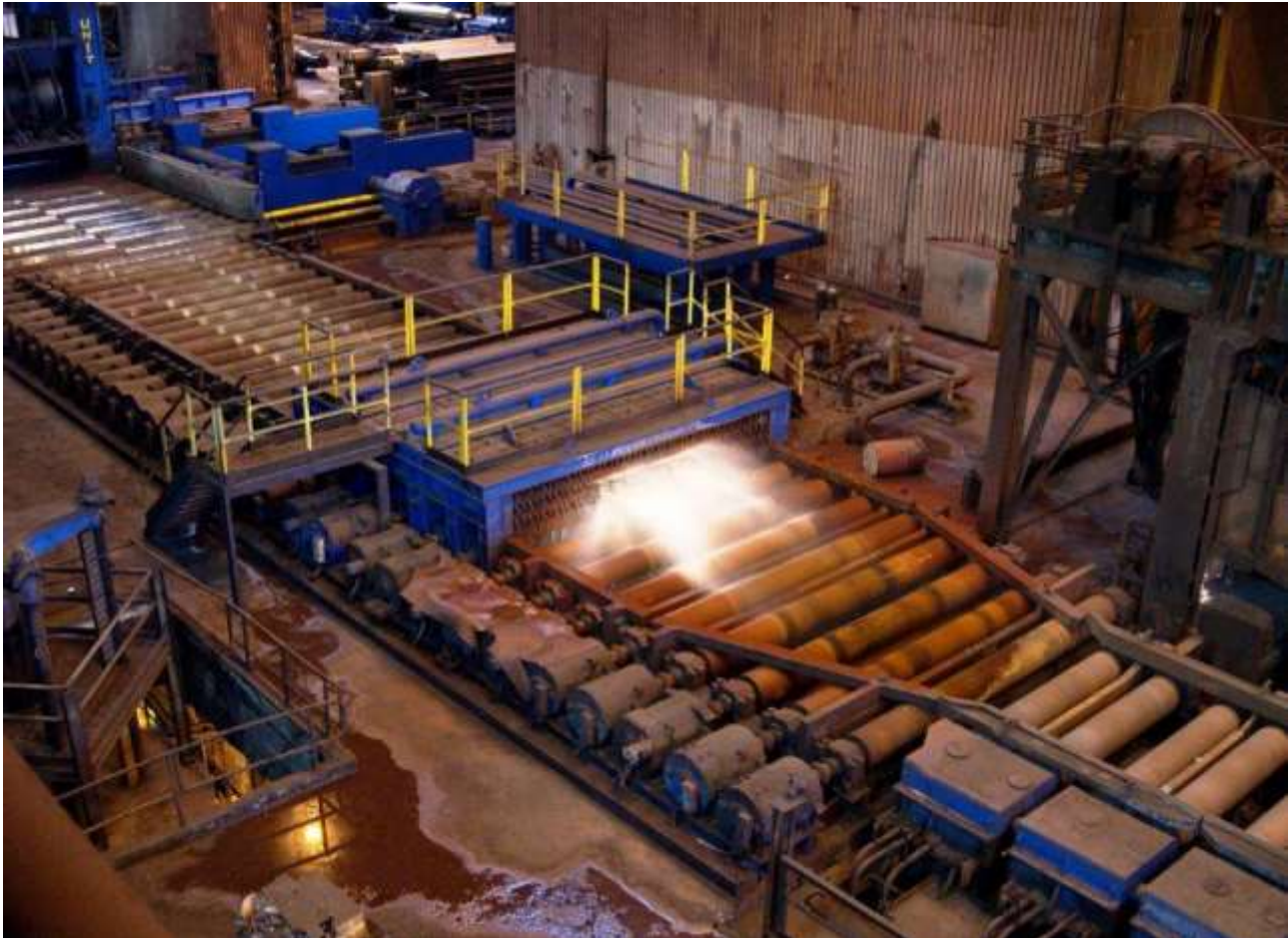
Revamping from furnace slab discharge to roughing mill (roller way, descaler, centring pushers)
