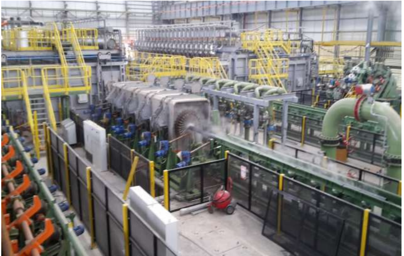
Detail of the quenching treatment zone
