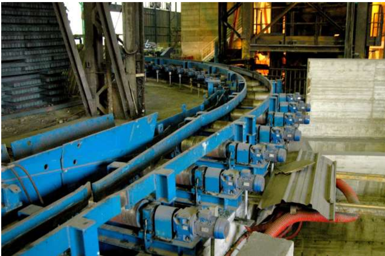
Curved roller way for billets, from reheating furnace to roughing mill stand
