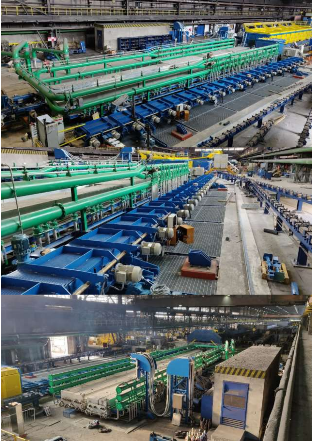
8-lines, 30 m tempcore and by-pass roller way
