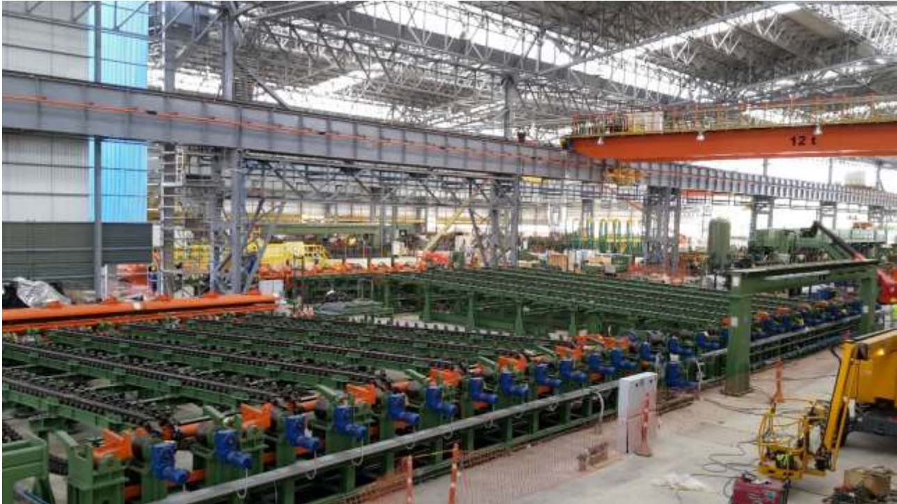
Quenching and hardening treatment plant for tubes during the erection
